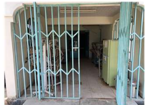
Entrance to CSRH operating ward construction site
